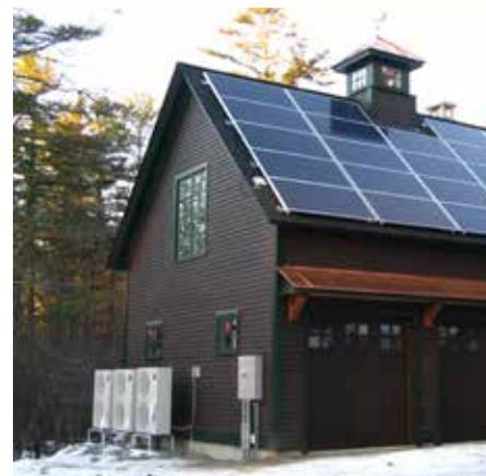
The heating system, installed and designed by ARC Mechanical Contractors, includes three Mitsubishi Electric MXZ all-weather air-source heat pumps.
