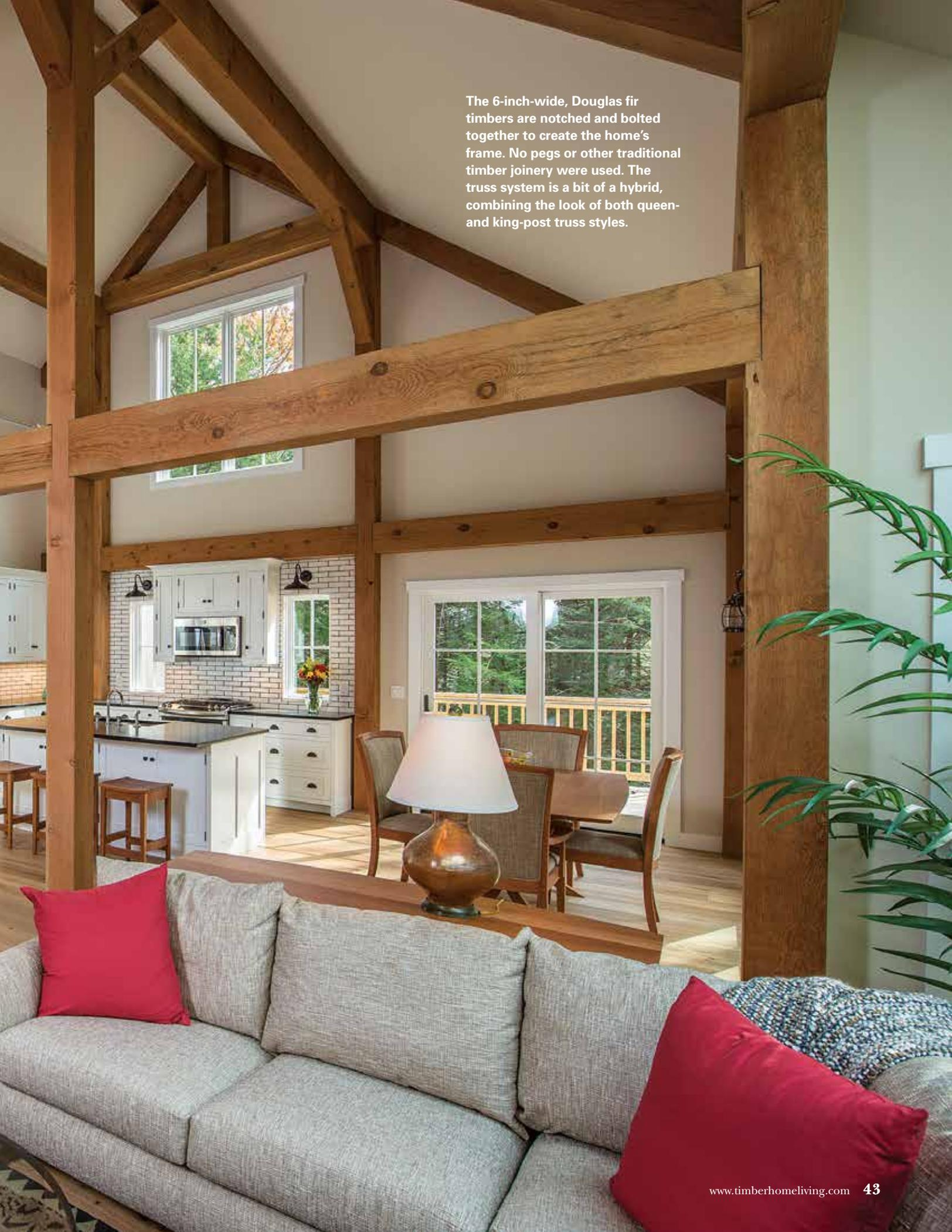
The 6-inch-wide, Douglas fir timbers are notched and bolted together to create the home's frame. No pegs or other traditional timber joinery were used. The truss system is a bit of a hybrid, combining the look of both queen- and king-post truss styles.
